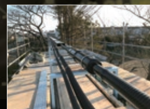
Three-phase coaxial superconducting cable system
